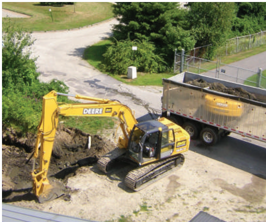
Contaminated soil excavation during remediation phase.
