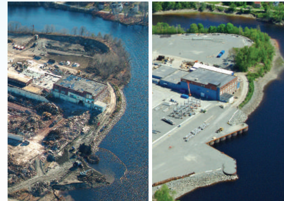
Site demolition, and site development complete.
